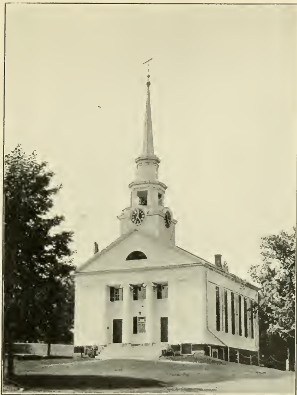
UNITARIAN CHURCH, CHELMSFORD CENTRE
